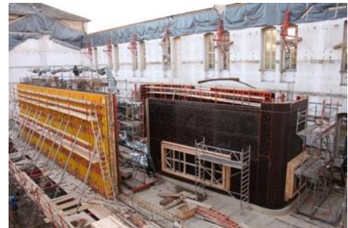
Abb. 6: Rohbau Hai Becken
